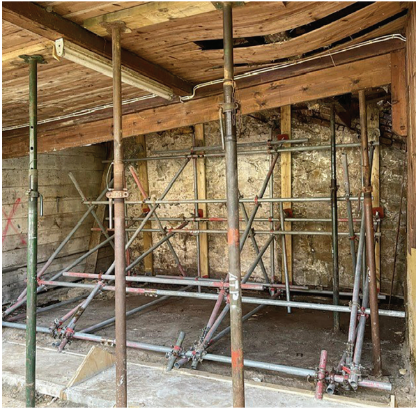
Interior view before restoration
