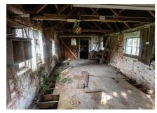
for like from materials reclaimed from elsewhere on the Estate. Cobbles removed from inside the building were reused at the thresholds, and new hardwood double glazed windows were designed to match the original fenestration.
